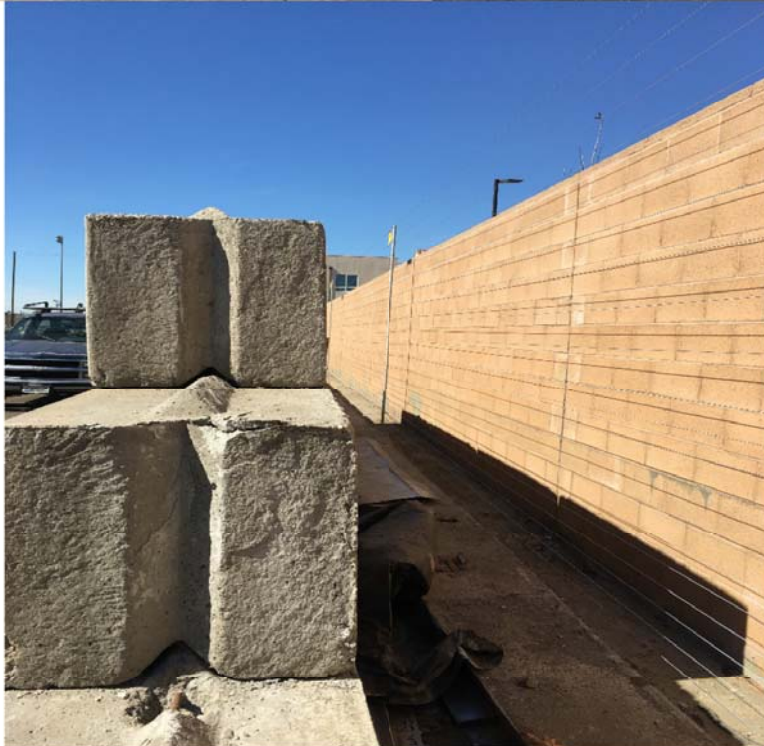
Photographs 1-3: Entrance to the northern side of the facility. The operator is installing a wall of concrete blocks to protect adjacent wall.
