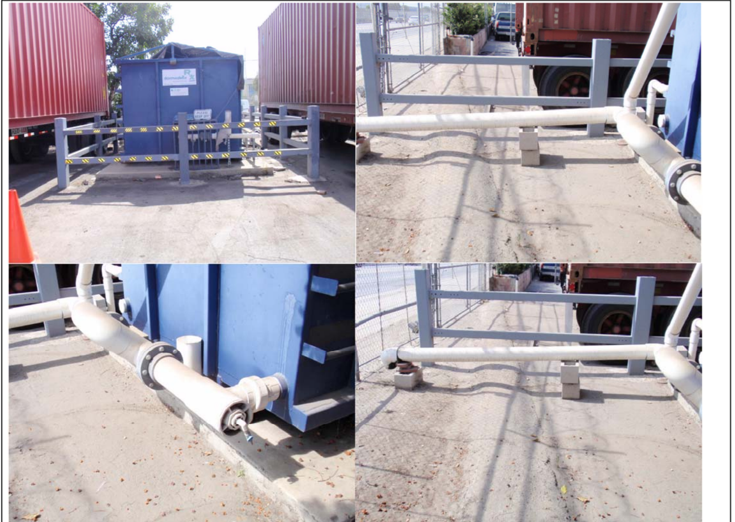
Photographs 38-41: The photographs show a storm water treatment system onsite, and a concrete berm placed along the north side of the facility to contain and re-route storm water to the treatment system.
